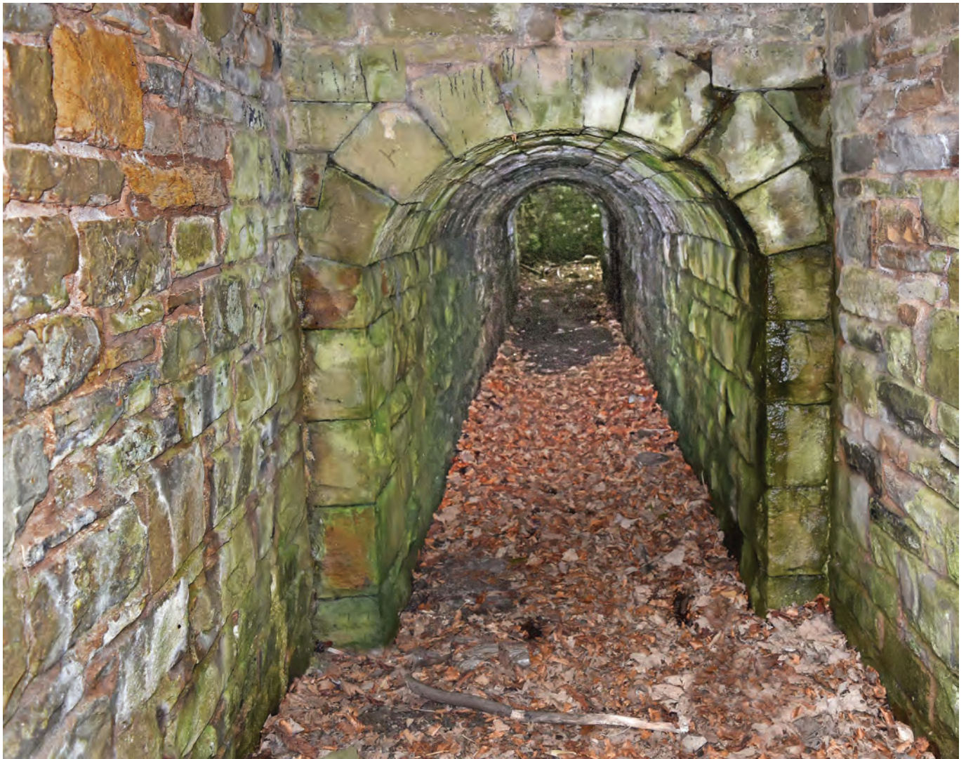
Inside the subway looking northeast towards Holme Hall
